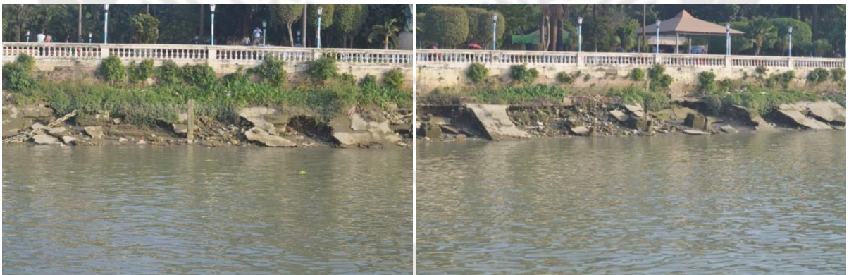
Fig.5A. Subsided, crumbled and dislodged bank at Millennium Park.
